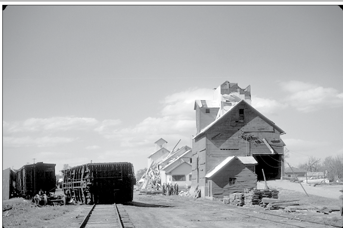
Hebron turns 150 years just four years shy of the May 9, 1953, tornado's 70th anniversary that crushed the city, claimed lives and split the Sacred Heart Catholic Church sanctuary. The photo above is taken from Lincoln Avenue looking north on First Street in front of the sale barn, and is from the collection of John and Idonna Kripal.
