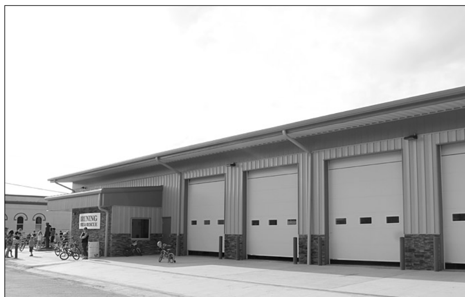
The new Bruning Fire and Rescue building opened its doors for the public during Bruning Days. Eighty to 90 donors contributed toward construction.
