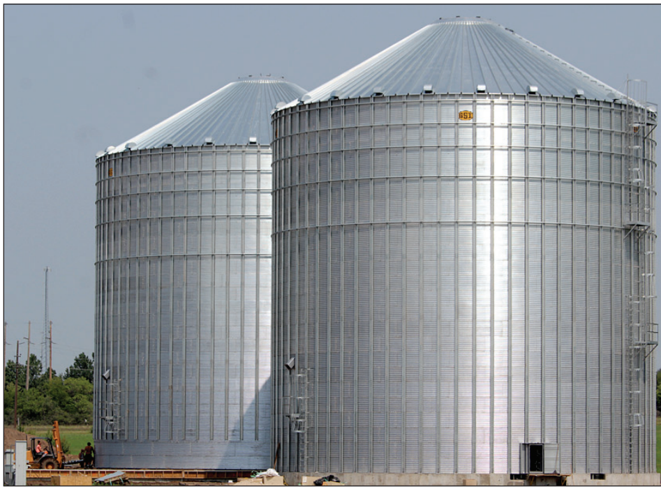
Norder's has added two grain bins. Construction is finishing up and the bins will be in operation in early October. Each bin will store 250,000 bushels to accommodate customers more efficiently and keep grain off the ground.
