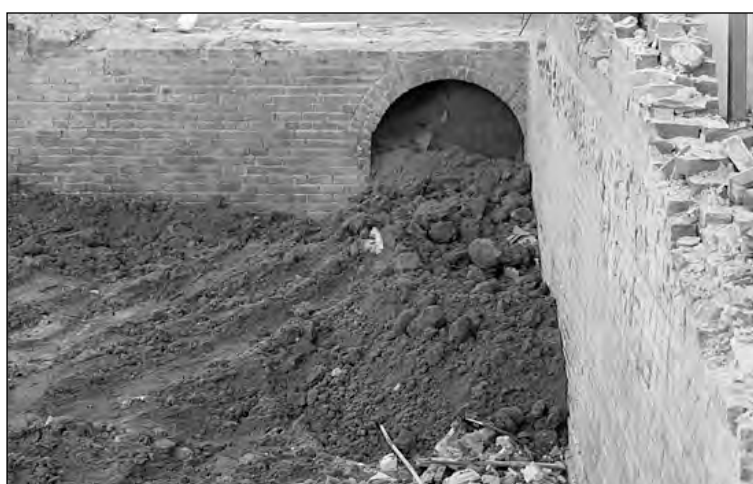
One of the projects the city council worked on in the past year were dilapidated buildings on 4th Street. The demolition is nearly complete. Once the hole is filled, which should be soon, the barricades on the street will be removed. The street and sidewalk will also be cleaned by the city.
