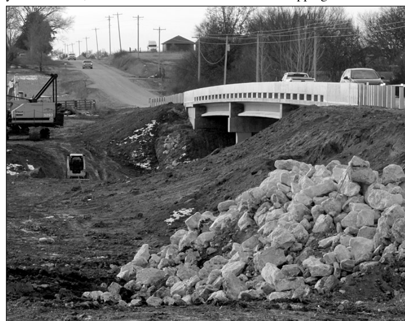
The First Street bridge opened last week after 18 months of closure because of flooding in May of 2015.
