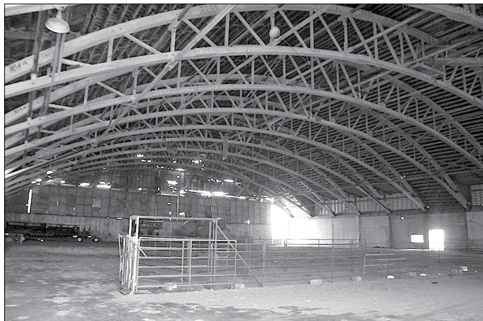
Inside the former World War II hangar that planes could fly right into, sits grain at harvest — Dan Domeier said he can store 600,000 bushels. The hangar was abandoned because the scale went bad, and it was sold to Domeier and his father, Darrel Domeier. On the north end of Domeier's feed yard is the old runway for the air base.
