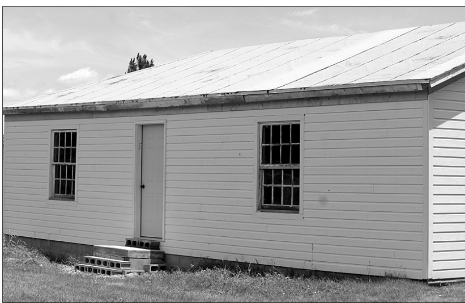
Bob Reinke, president of the Thayer County Museum and Historical Society, moved a Civilian Conservation Corps/Prisoner of War building from Hebron to the Thayer County Museum grounds. He thinks the building may have been part of a larger structure. It has received new paint and siding, and is currently receiving a new floor, however, Reinke said the inside shows the mismatched boards used to build the structure as they were sometimes hastily constructed. Military items will most likely be stored inside once its completed. Reinke has personal ties to the POW era, in which prisoners were housed in Hebron from 1943 to 1945, and hired by local farmers. Reinke's grandfather hired POWs to work in the fields near Byron and became good friends with them.
