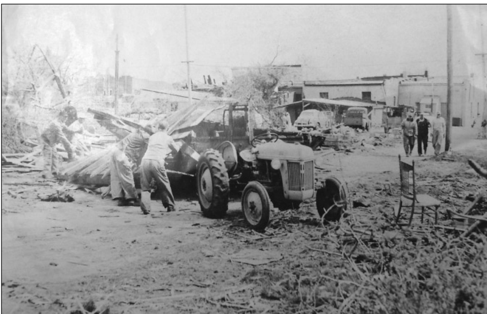
On Monday morning the work of cleaning up began in earnest. Volunteer workers began to pour in by the dozens with trucks, tractors, dozers and all types of hauling equipment. ~The Hebron Disaster~
