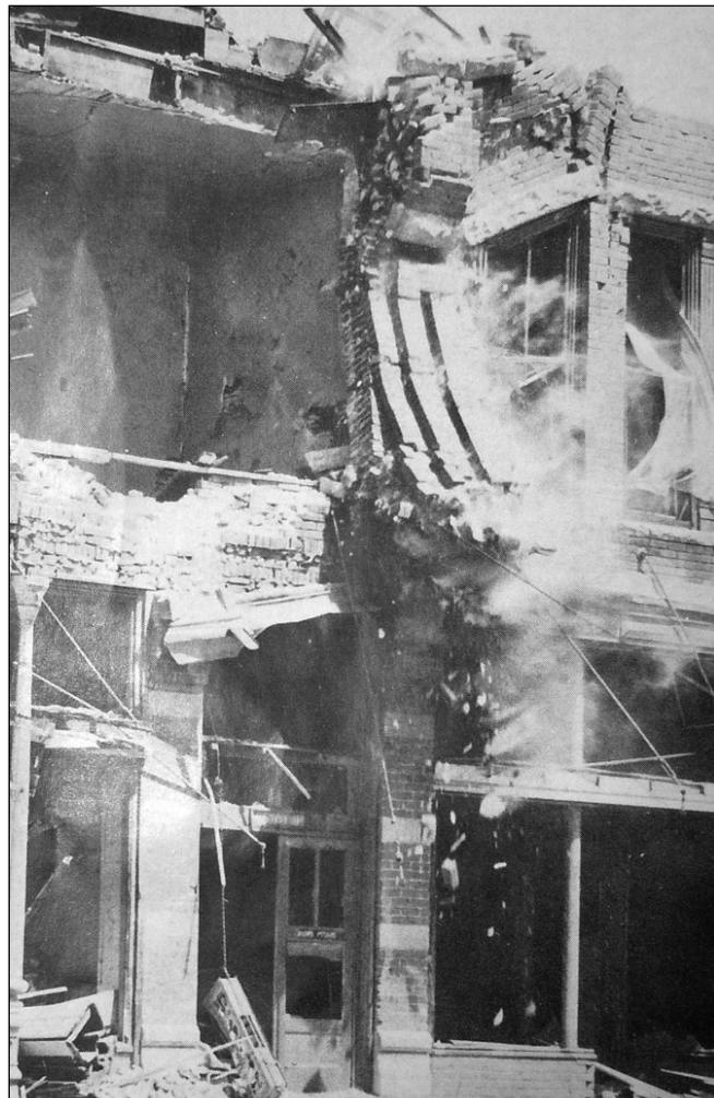
Several building fronts that were damaged by the storm had to be pulled down by cable trucks for the protection of the citizens and workers. ~The Hebron Disaster~
