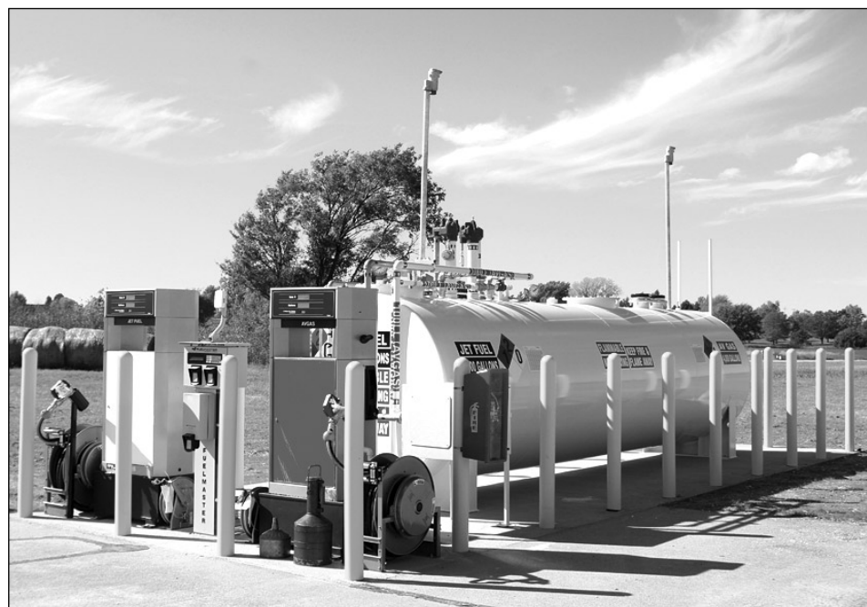
A new 5,000-gallon split fuel tank at the Hebron airport that accepts credit cards will be in service Nov. 3. The tank has 1,000 gallons of Jet A and 4,000 gallons of 100LL.
